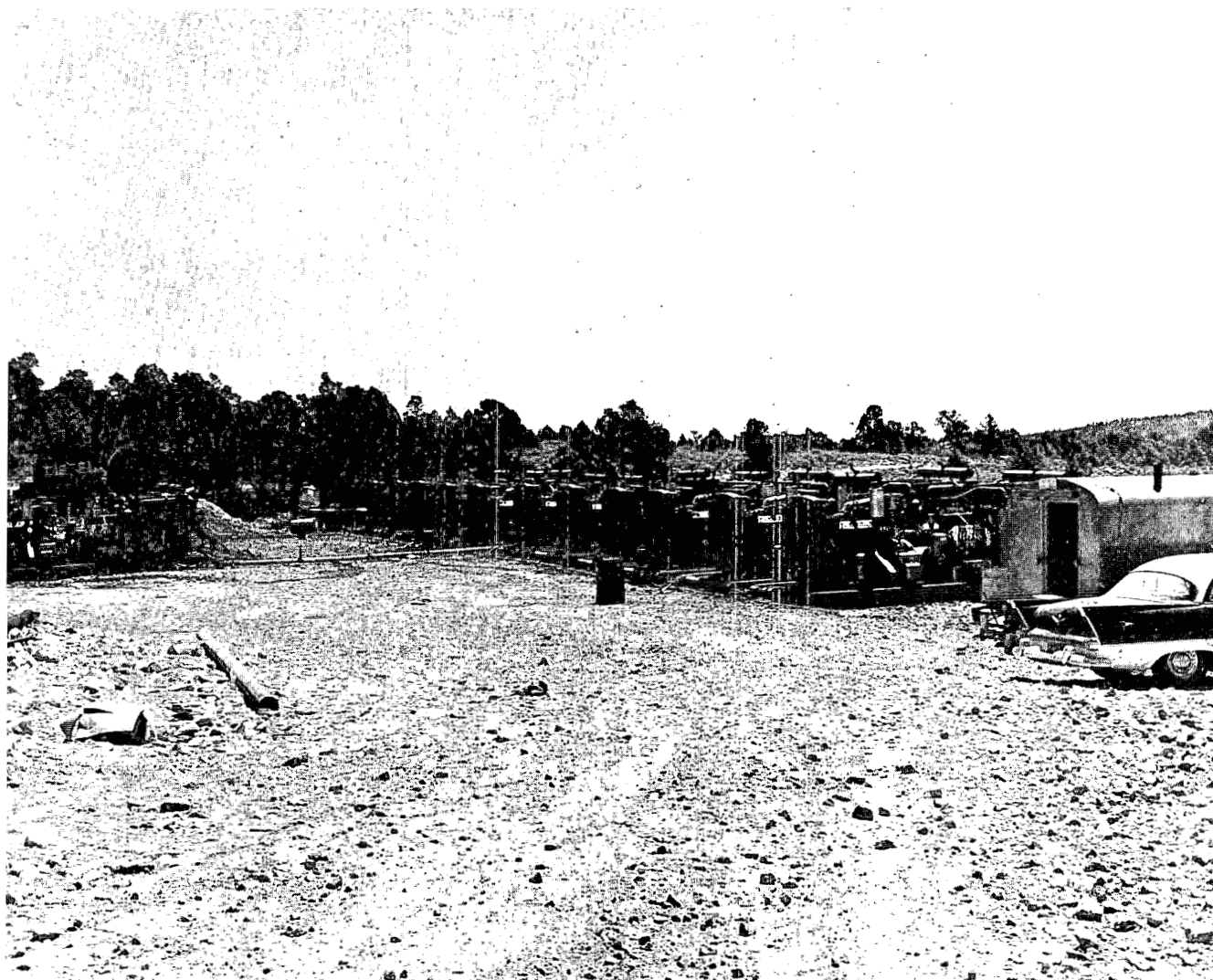
Fig. 16. View of a bank of air compressors being used as the air supply for direct air circulation on a 64" diameter hole. Photo-USAEC.
